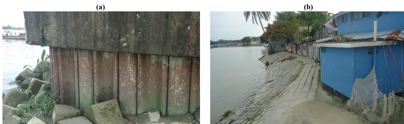
Figure 3. Representative physical structures of the PTPE project: (a) steel sheet-pile floodwall with concrete capping and toe protection; and (b) riverbank revetment adjacent to residential development. Source: field photographs taken by the authors.
