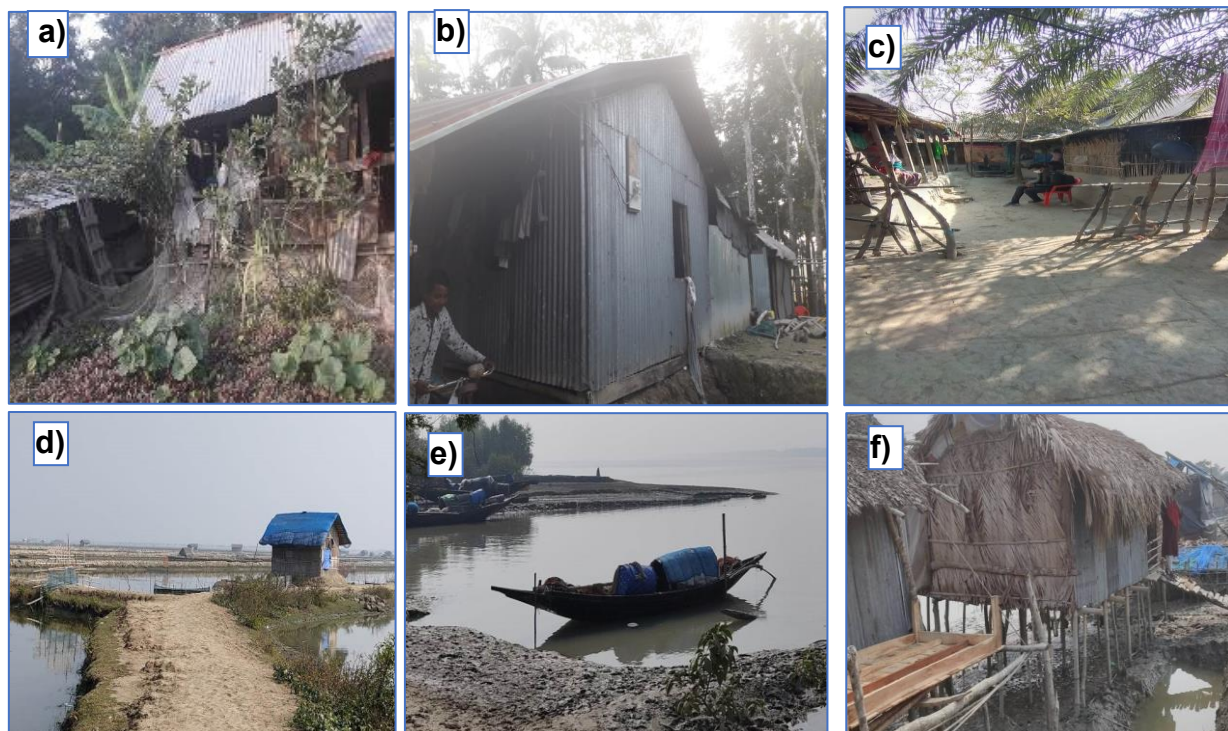
Figure 7. Some ideal pictures showing the vulnerable and fragile structures (a,b,c) vulnerable houses (d) earthen and fragile embankment and (e, f) houses adjacent to the river system. Source: authors.
